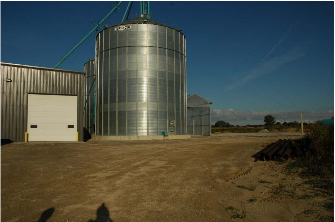
Figure 1 Fuel Storage Siloes at Southshore Greenhouses with Covered Truck Unloading to the Right
